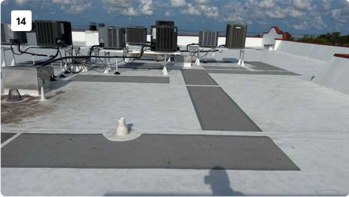
Roof Level Images
