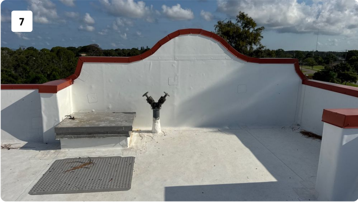
Roof Level Images
