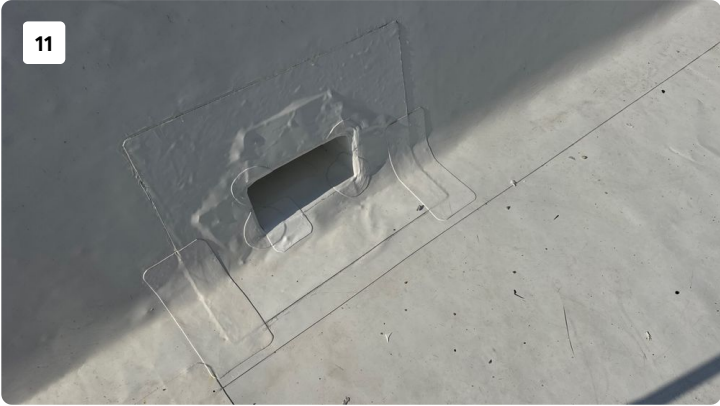
Roof Level Images
