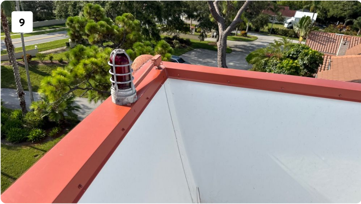
Roof Level Images
