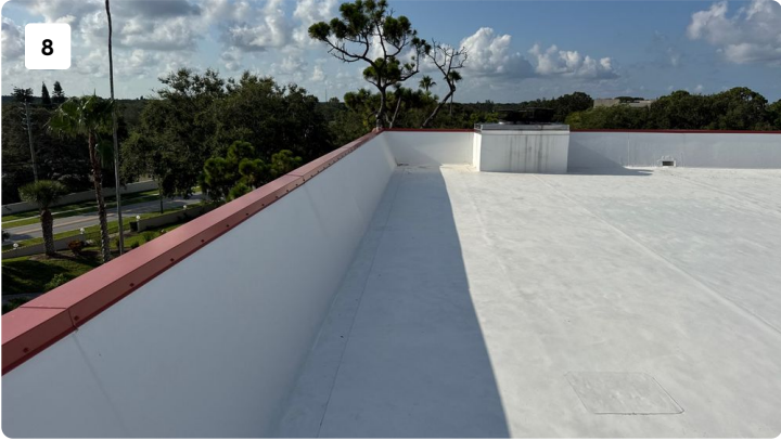
Roof Level Images
