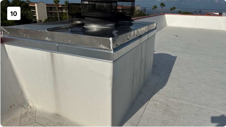
Roof Level Images
