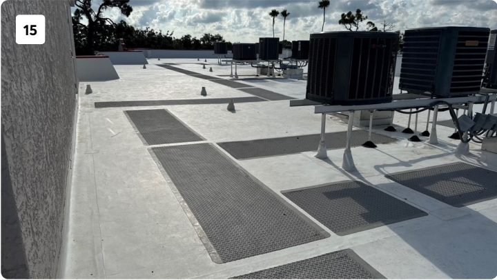
Roof Level Images
