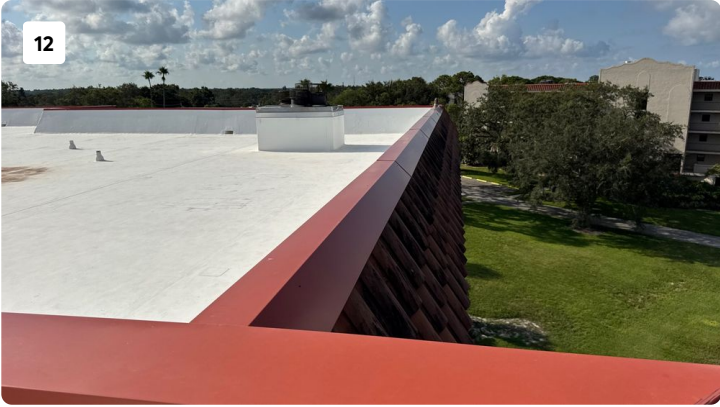
Roof Level Images
