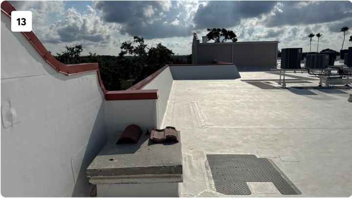
Roof Level Images
